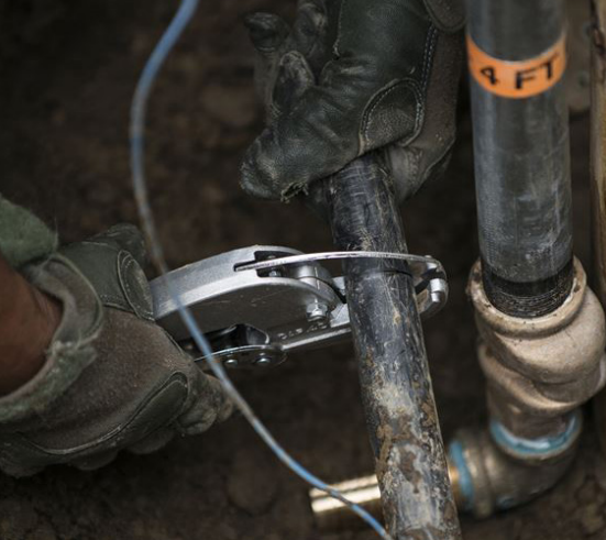
Lead Service Line Replacement
