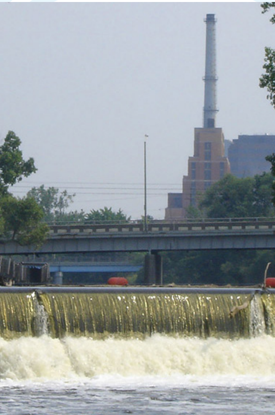
North Lansing dam
