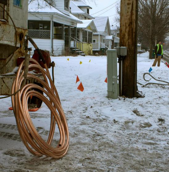
A copper service line will replace a lead service line on this residential street in Lansing. In the background is a lead service line that's been removed. *Image taken and courtesy of Lindsey Scullen of Michigan Radio*
