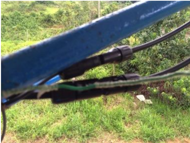
Figure 2. Two MC-4 connectors
