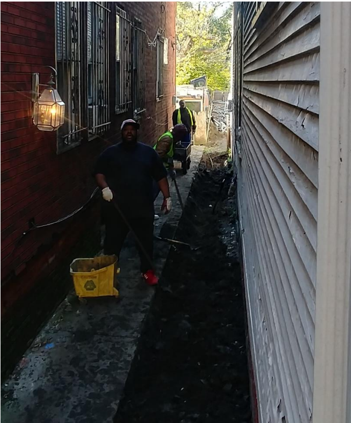
Volunteers at Hubbard, digging a swale to remediate water logging around the foundation
