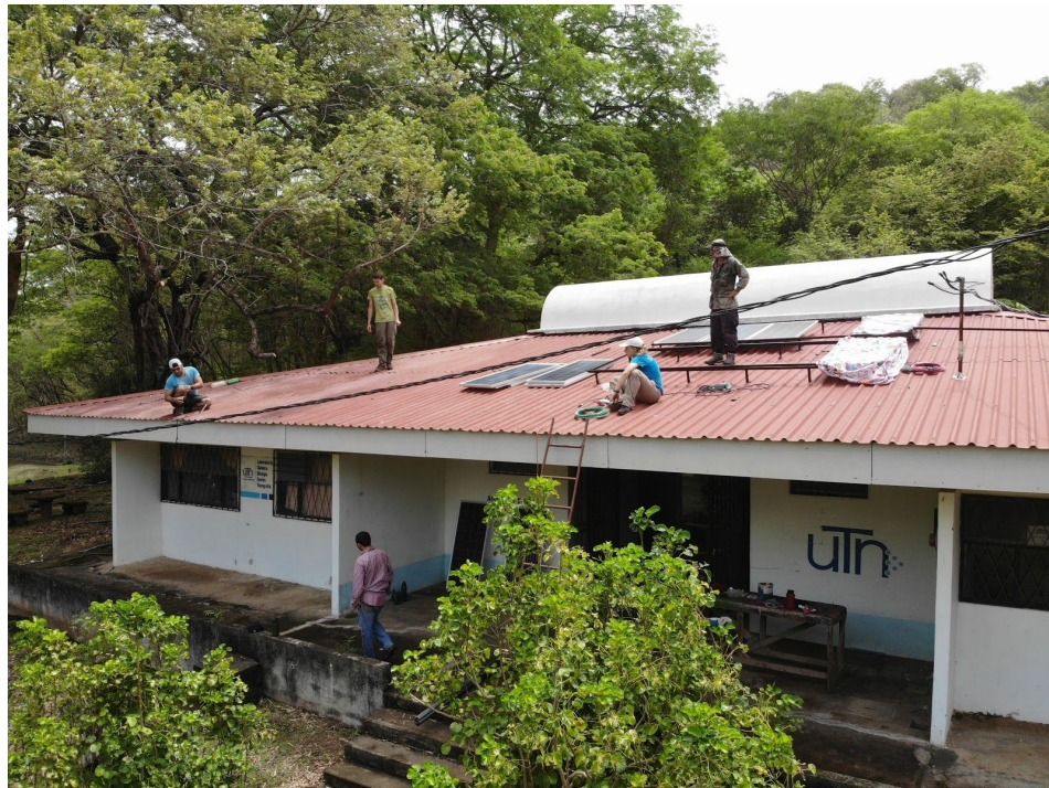
Picture 1: solar array being installed
