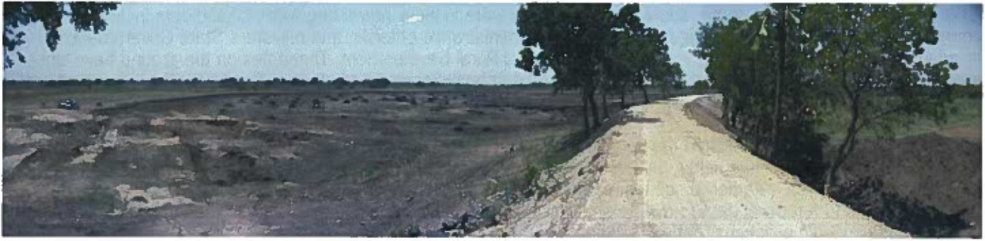
A de-silted pond and the rebuilt berm. Warangal, Telangana
