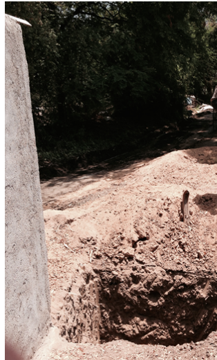
Figure 2: The outhouse is on the left and the pit for the septic tank is on the right.
