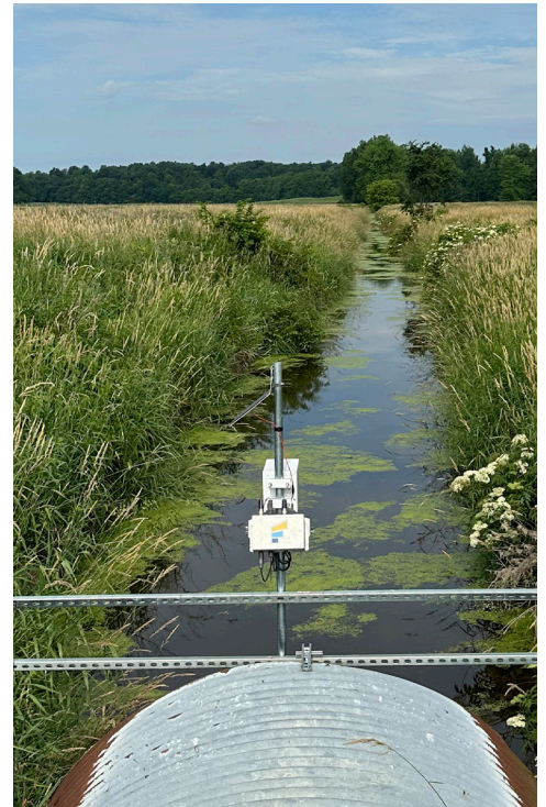
Water quality monitoring equipment in an agricultural ditch in Lenawee County. Photo: Fatimah Bolhassan
