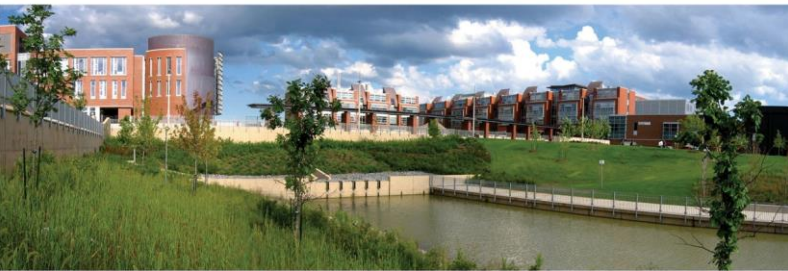
Storm Water Retention Pond
