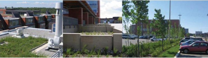
Roof Gardens & Parking Lot Bio-swales
