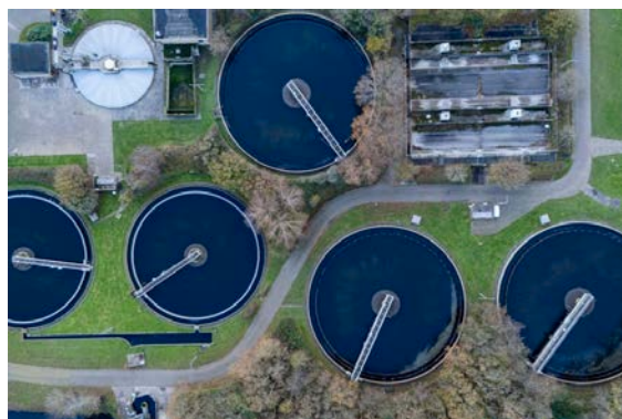
Clarifier tanks at a wastewater treatment plant
