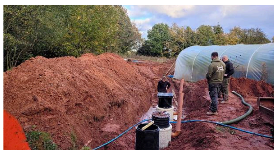
Septic tank installation. Photo: Jonathan Billinger, CC BY-SA 2.0, via Wikimedia Commons
