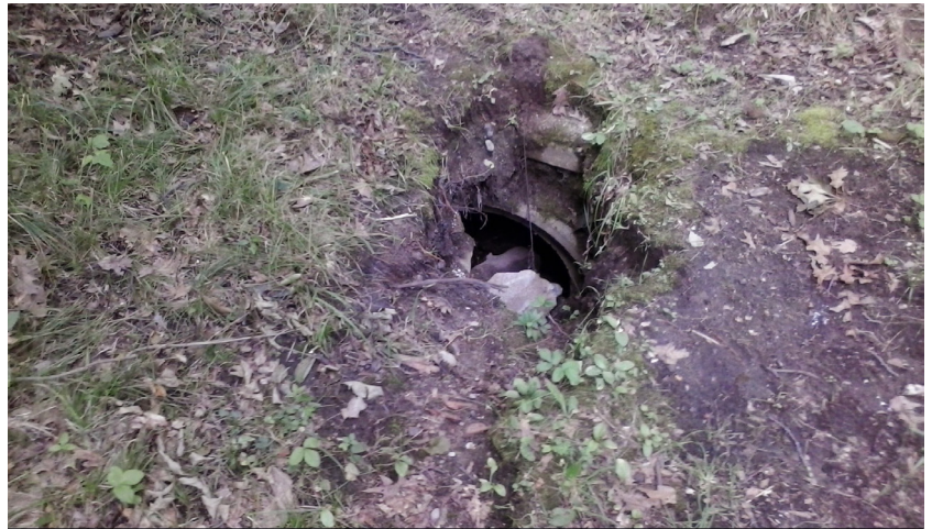
Before Project Work: Broken Culvert
