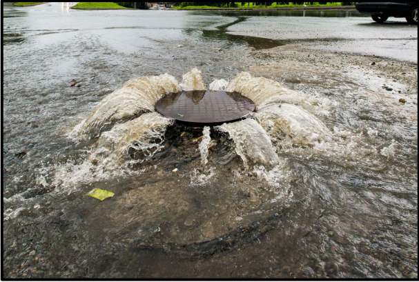
Sanitary Sewer Overflow (SSO)
