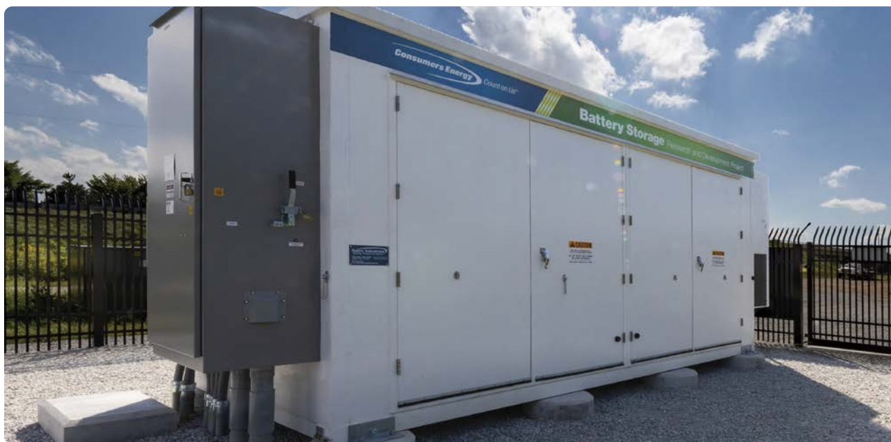
The 1 MW Parkview Battery Project on Western Michigan University's campus in Kalamazoo is the first lithium-ion BESS in Michigan. (Photo: Consumers Energy)
