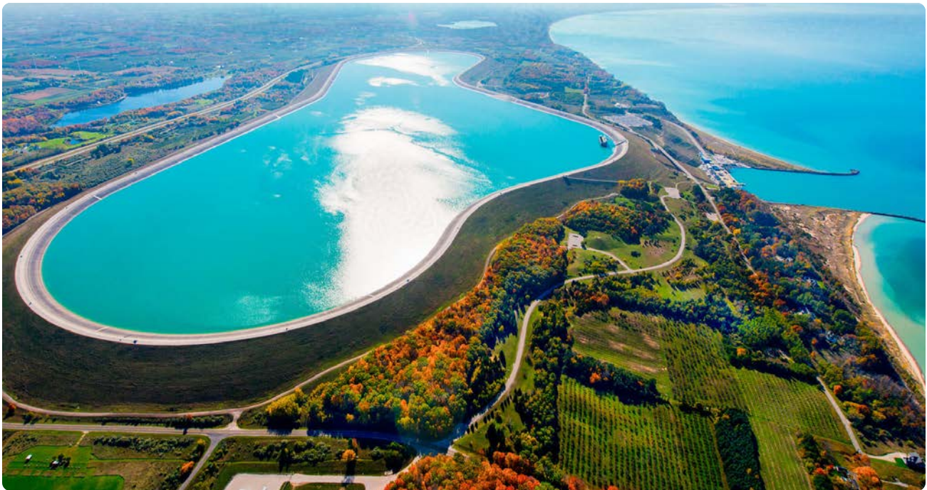
With a capacity of 2,292 MW, the Ludington Pumped Storage Plant is located on a 1,000 acre site along Lake Michigan. It is jointly owned and operated by Consumers Energy and DTE Energy. (Photo: Consumers Energy)
