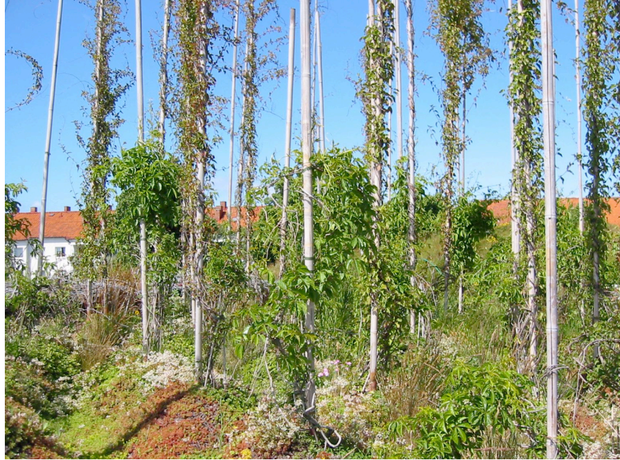
Figure 2.7 An example of a semi-intensive green roof in Augustenborg, Sweden (photograph by Andrew Turner).
