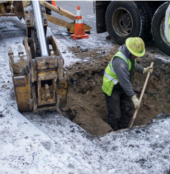
A crew member continues to dig toward one of Lansing's lead service lines. Image taken and courtesy of Lindsey Scullen of Michigan Radio
