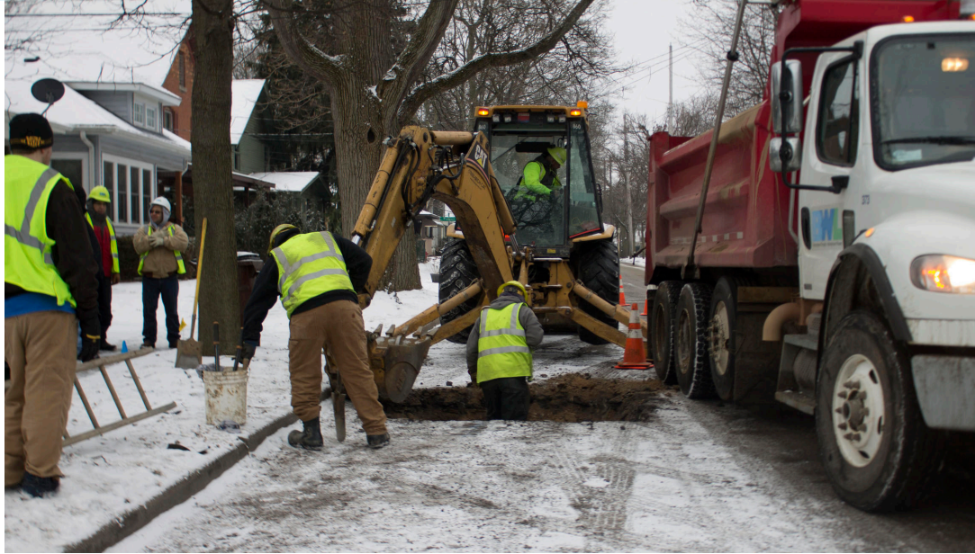
Crew members in Lansing get closer to the lead service line they plan to remove. Image taken and courtesy of Lindsey Scullen of Michigan Radio
