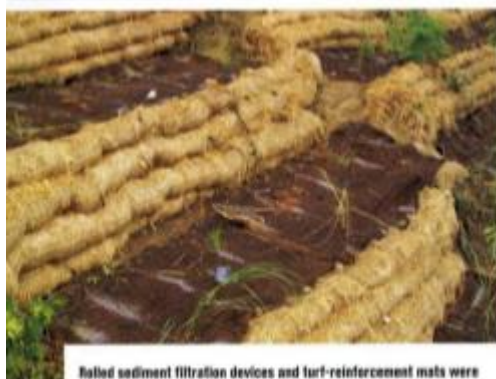
Rollled sediment filtration devices and turf-reinforcement mats were used to build and stabilize the terraces.
