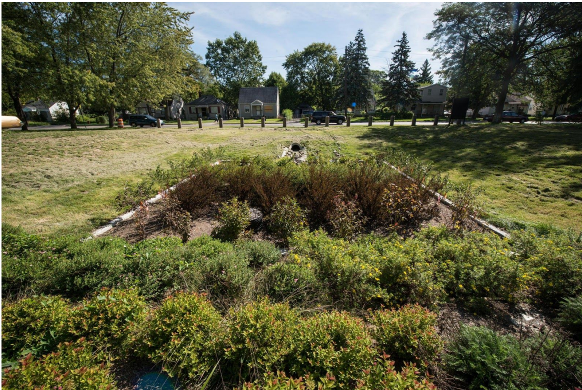
Figure 1: A bioretention garden manages stormwater in the Warrendale neighborhood of Detroit. 1
