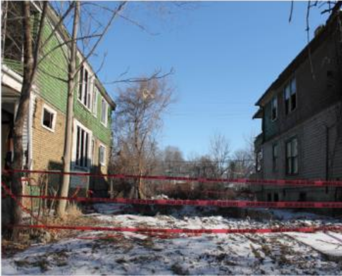
Demolition in progress
