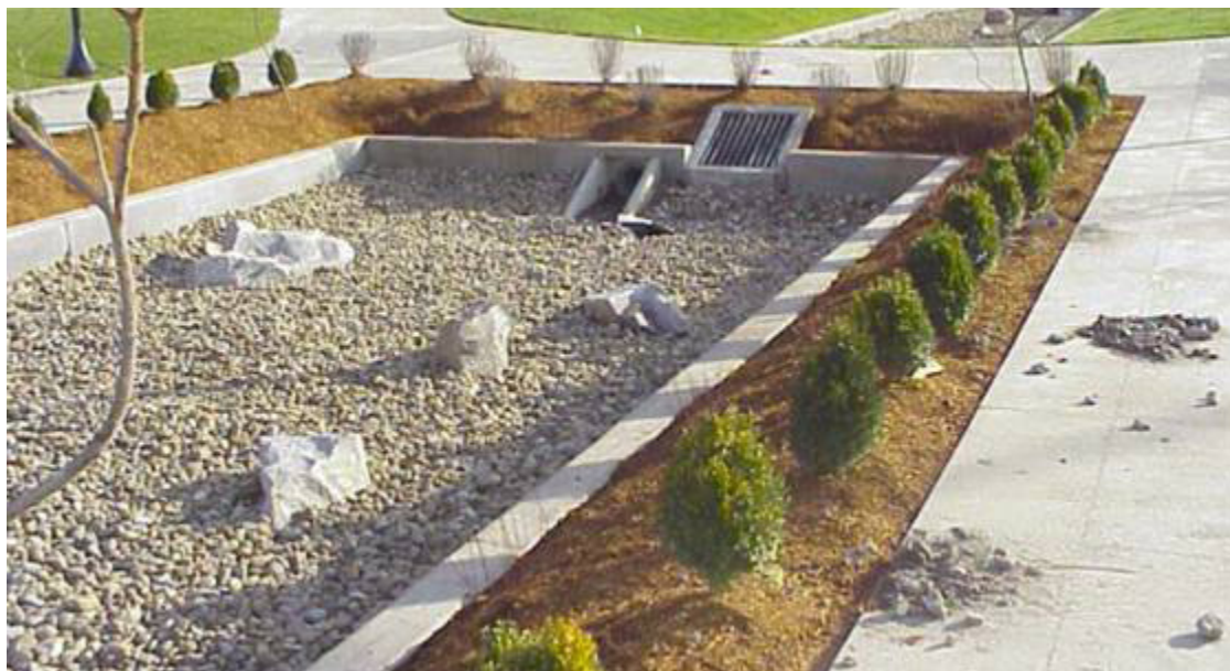
Figure II-4. A sand filter is an example of a Category A Quality stormwater management practice because it removes pollutants from the water through both sediment removal and filtration D
