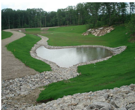
Figure II-3. A detention pond would be one of many stormwater management practices eligible for a quantity credit. c
